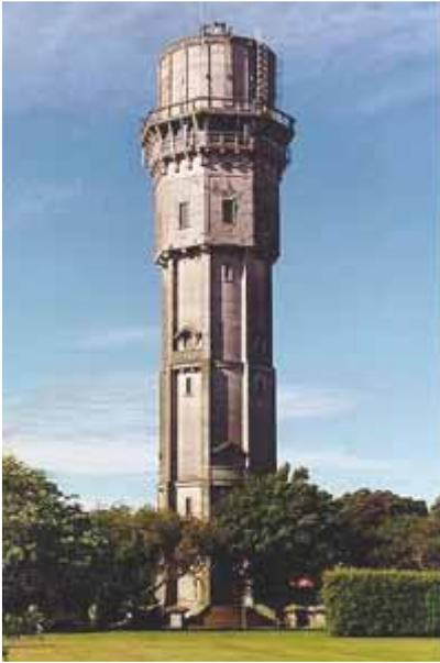
Where there is no high ground, water towers can be used to give the desired elevation. Water towers are no longer common for larger water supplies in New Zealand because of the expense in meeting earthquake safety requirements and the visual impact of these structures. Pressure-sustaining pumps are now a more usual solution. However, for water supplies serving a small population, water towers may still be cost-effective.
