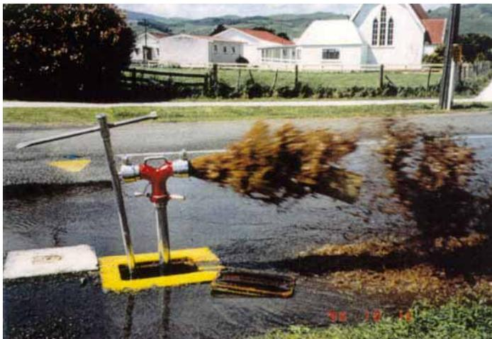
Care needs to be taken to ensure the flushing does not simply move dirt and contaminants around the system while clean water is discharged through the fire
